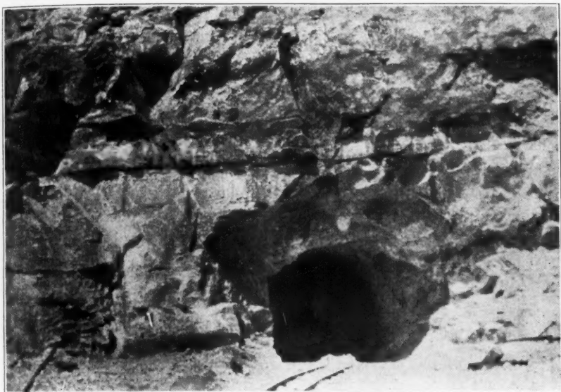
Tunneling to Get Away from Winter Weather
